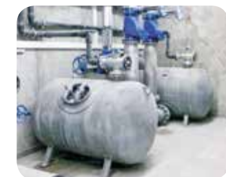
GULLICOMB® - The combination of the advantages of the hydraulic and pneumatic waste water transportation.
