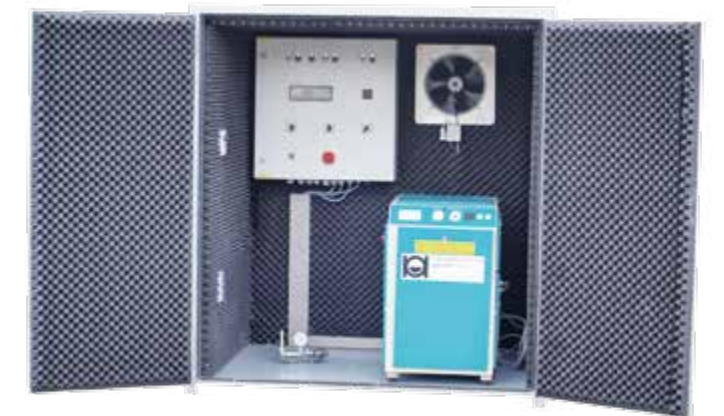
Concrete equipment cabinet with a 7.5 kW screw compressor and an integrated pump control
