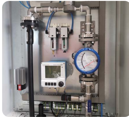
Regelung Neutralisation Neutralization control
